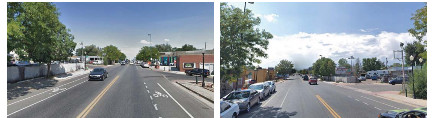
Existing S. Meade St. and Morrison Road intersection
