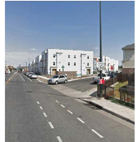
Existing W. Ohio Ave and Morrison Road intersection.
