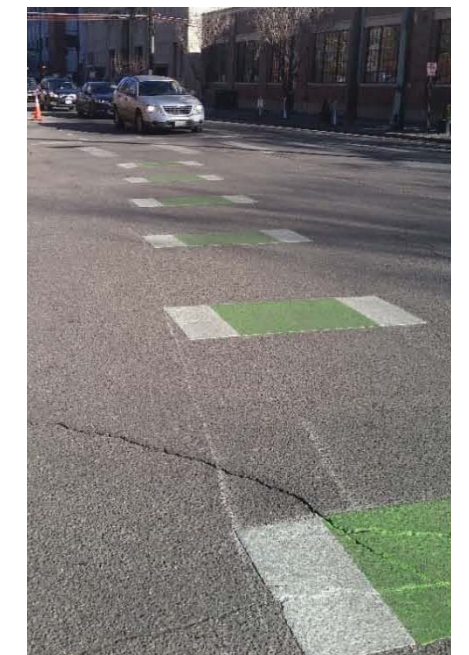
Figure 9: Green Pavement Markings for Bicycle Intersection Crossing: Denver
