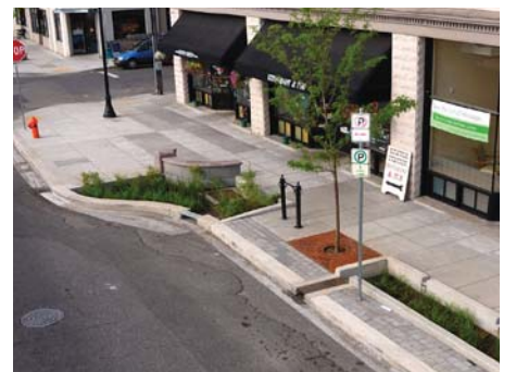
Planters with integrated seating; Stormwater Streetside planters
