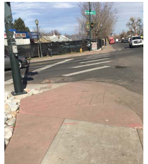
Existing pedestrian crossing at W. Kentucky Avenue and Morrison Road
