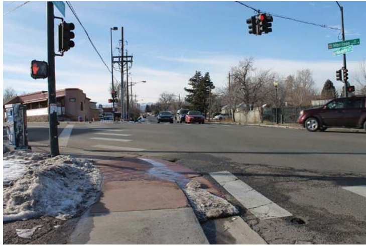
Existing W. Kentucky Avenue and Morrison Road intersection
