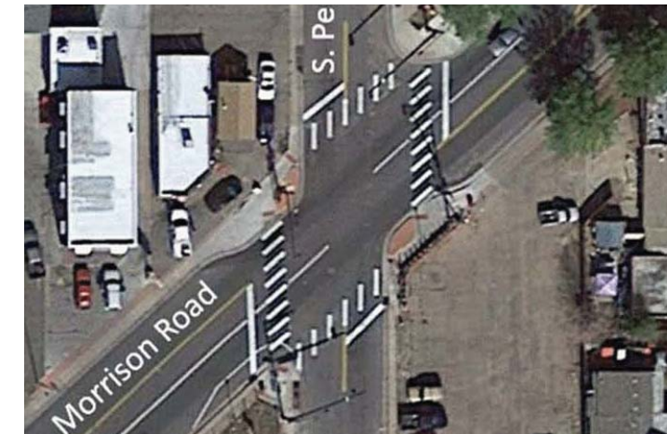
Figure 3: Morrison Road at S. Perry Street - Existing Configuration (Google Earth)
